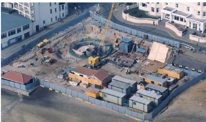
Extensive alterations taking place in March 2000.
